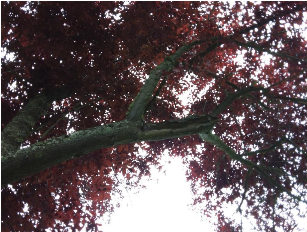
Figure 9. Photo of breakout point with associated decay.
