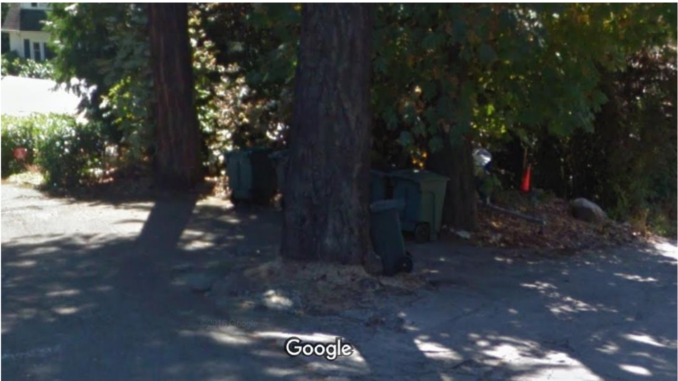
Figure 17. Close up of the bases of the three firs showing how the pavement wrapped around the trees. Note the distance that the edge of the road is from the #1 fir.
